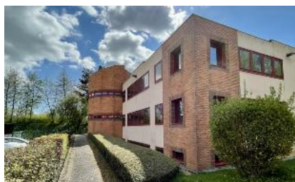
- BOIS GUILLAUME - Location & Vente 720 m 2
